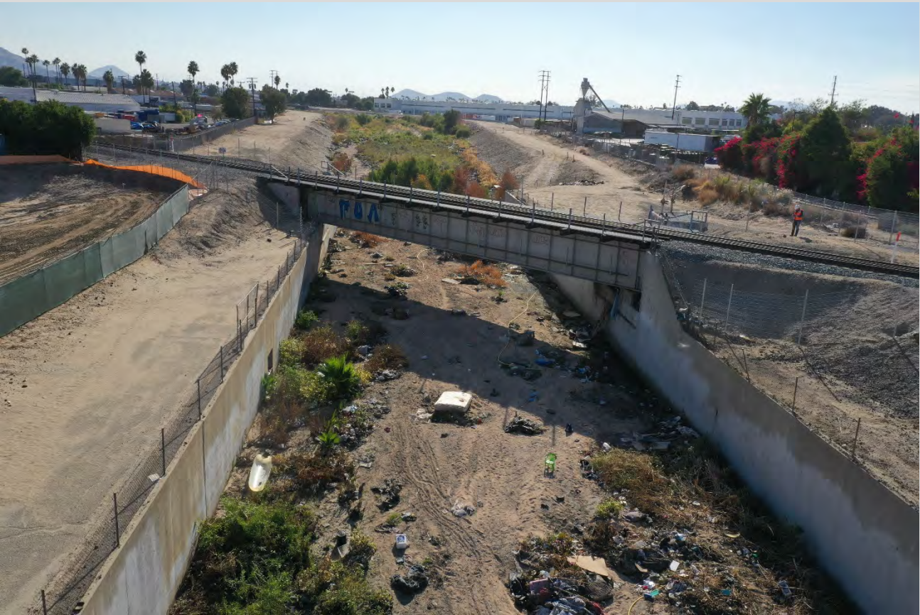
Twin Creek Bridge - October 2021
