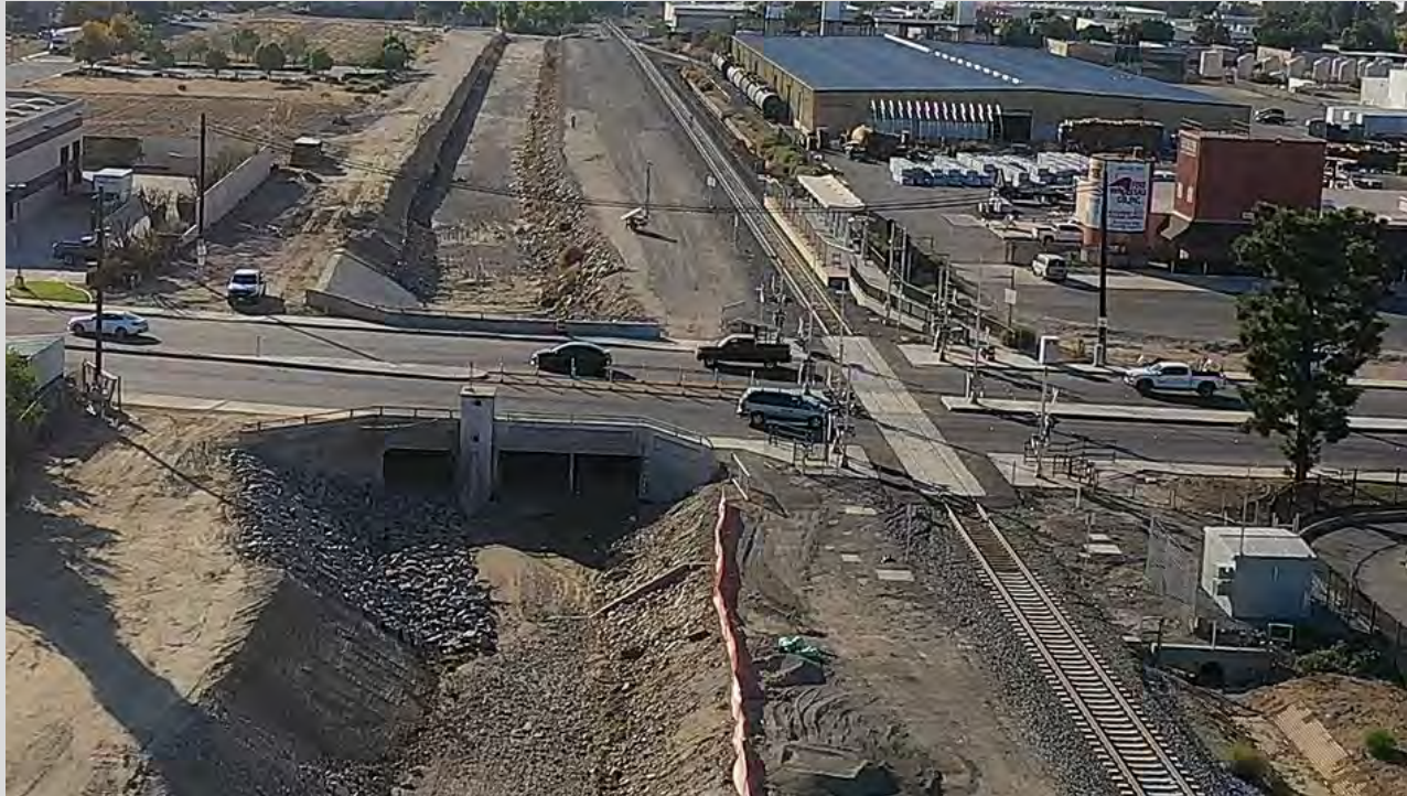
Tippecanoe Avenue Road Crossing - October 2021
