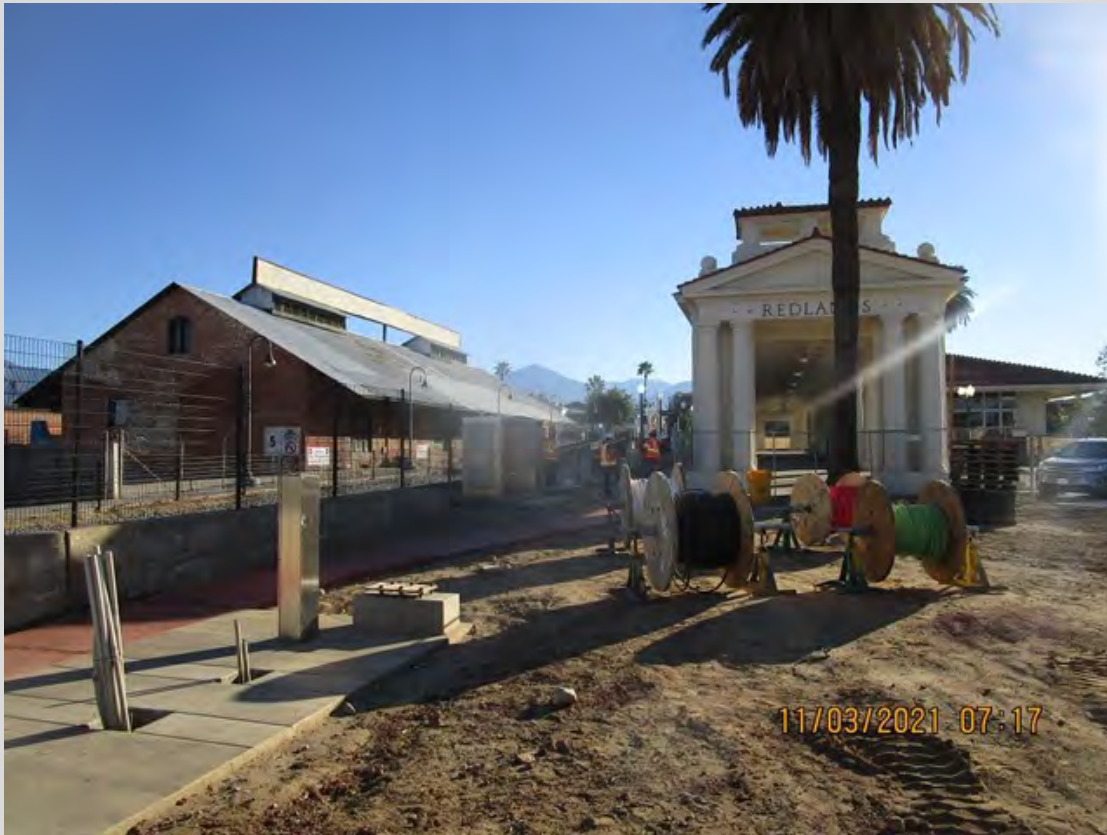
Contractor Pulling in Wires at Redlands - Downtown Station - November 2021
