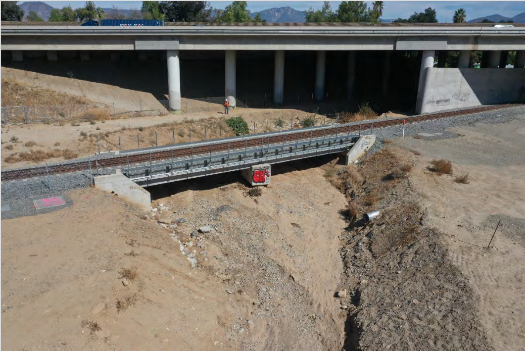
Mill Creek Zanja Bridge - October 2021
