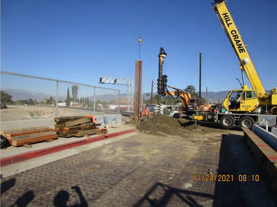
Mountain View installation of #5 shoring pile - November 2021
