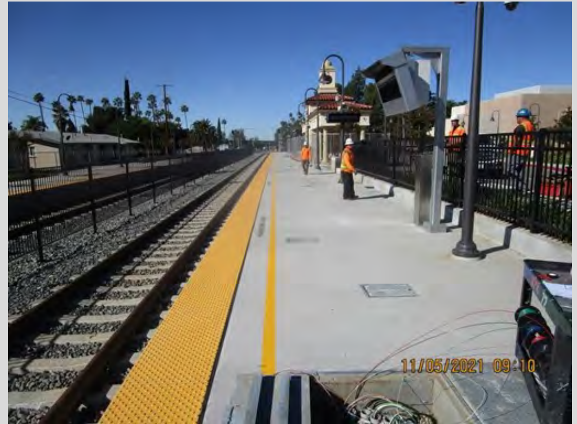
Contractor Pulling Wires at University Station - November 2021
