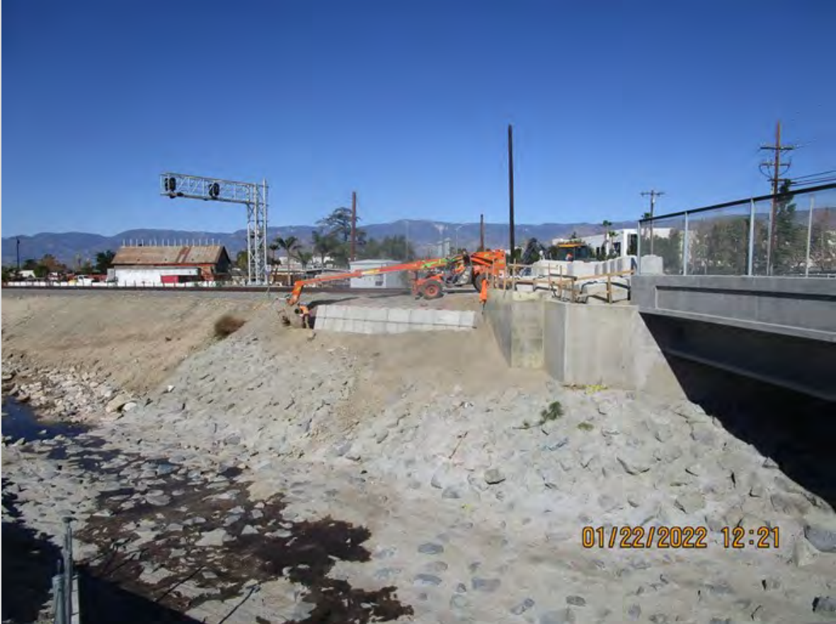
Installation of 2nd block wall at Mountain View - January 2022
