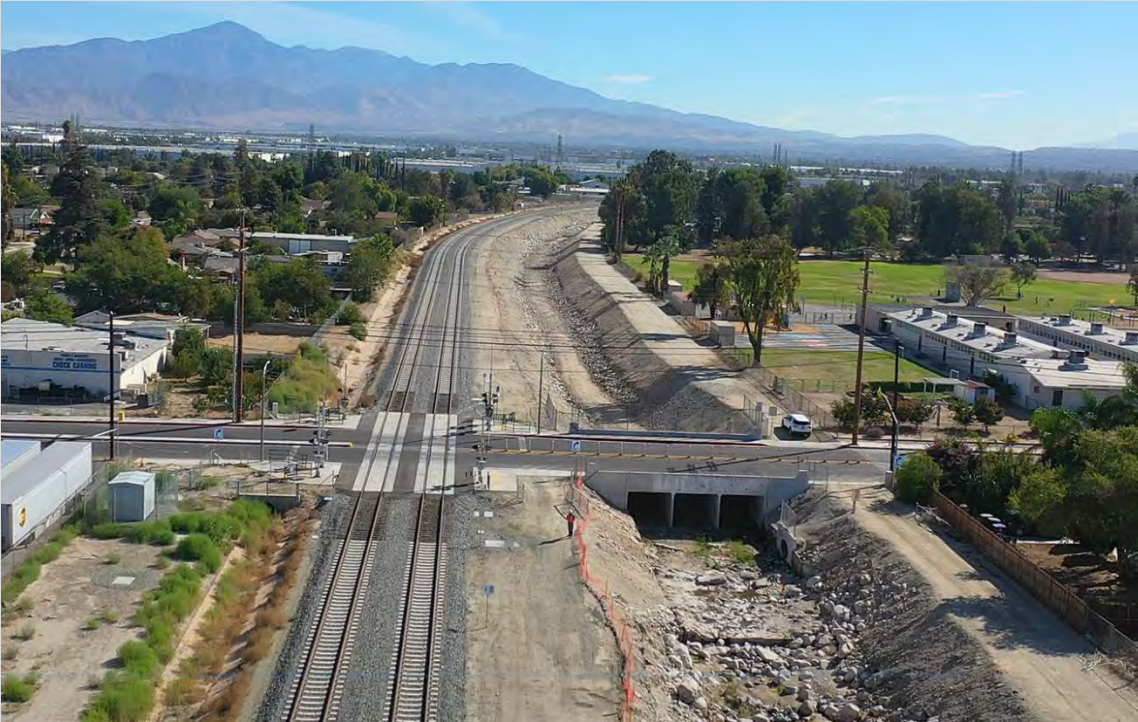
Richardson Avenue Road Crossing - October 2021
